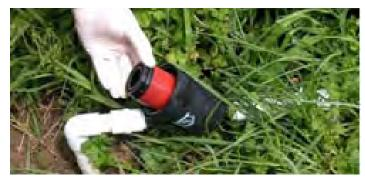
8. Screw up top of filter housing by hand until securely tightened.
